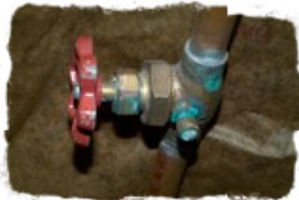
1. Locate your water faucet shutoff valve. Mine is located in my basement above the drop ceiling. It's about four feet in from the basement door. If you have a finished basement with a drop ceiling you'll need to get a step ladder and move a ceiling tile or two to locate it. It will look like the photo below.
