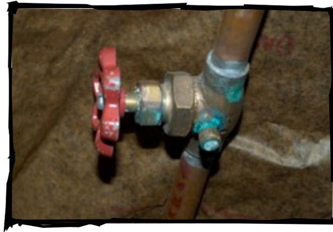
2. Turn off the shutoff valve. Make sure the valve is fully closed (turn clockwise to close), but don't over-tighten the shutoff valve.
