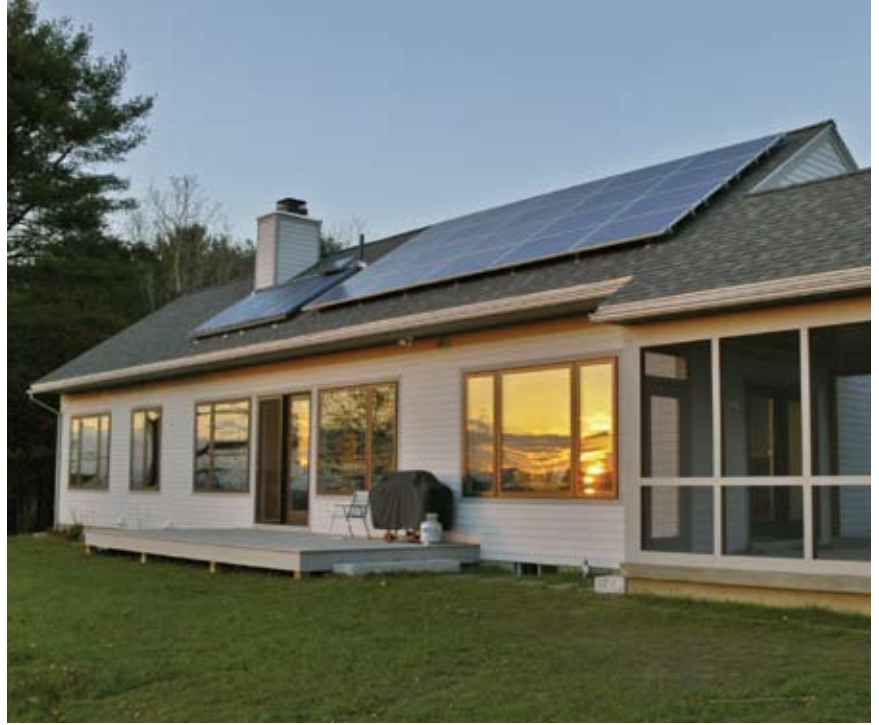
PV array in Amherst, MA
