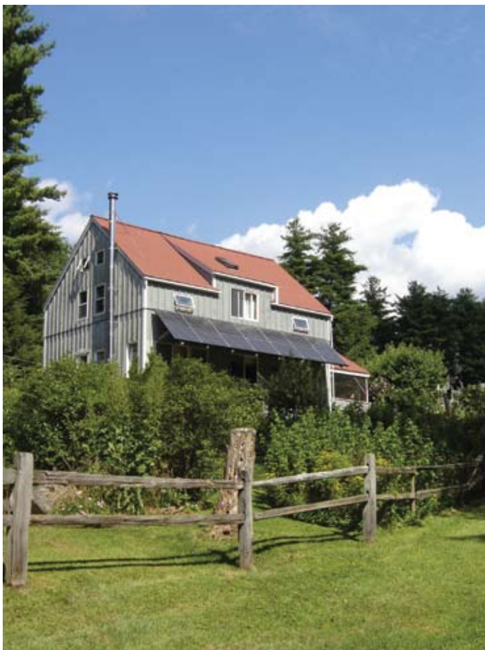
PV array in Great Barrington, MA
