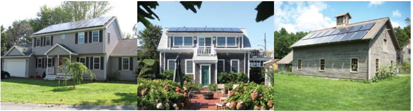
Left to right: Joyce residence's 6.3-kW PV array, Tewksbury; Hochman residence's 3.28-kW PV array, Provincetown; Piasecki residence's 2.4-kW PV array, Stockbridge
