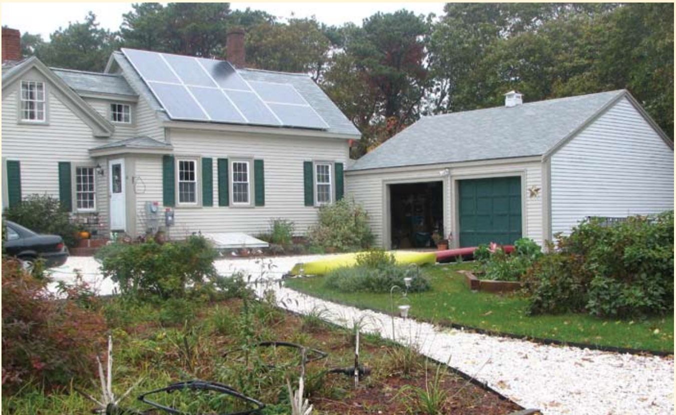
The Kemprecos house with rooftop PV
